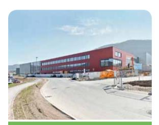
The new plastic housing module factory in Dettingen/Erms was designed to be as energy-efficient as possible. The production area covers nearly 20,000 m². A 450 kW photovoltaic system was installed over approximately 3,000 m² of the roof space. Heat from the machinery and equipment is used to warm the factory space and offices, thus saving around 1,300 MWh of primary energy per year.
