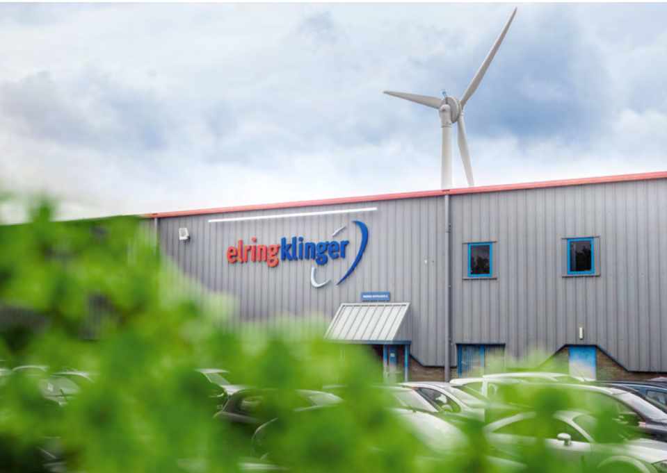
The wind turbine in Redcar generates approx. 1,400 MWh of green electricity at an average wind speed of 6.1 m/s. This saves some 600 tons of CO 2 a year.
